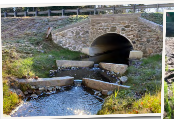
The Fish Habitat Program worked with NH Department of Transportation to design and construct a fish weir under Rt. 115 in Jefferson to ensure that wild brook trout can swim upstream to spawn in the headwaters of this stream.
