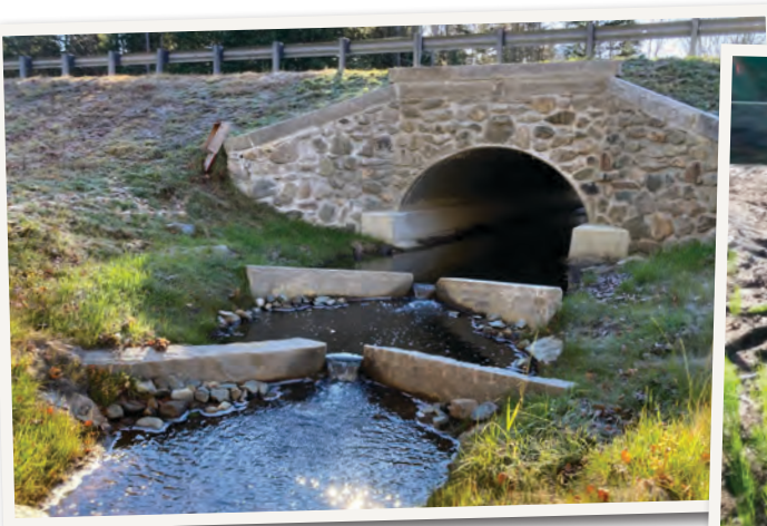
The Fish Habitat Program worked with NH Department of Transportation to design and construct a fish weir under Rt. 115 in Jefferson to ensure that wild brook trout can swim upstream to spawn in the headwaters of this stream.
